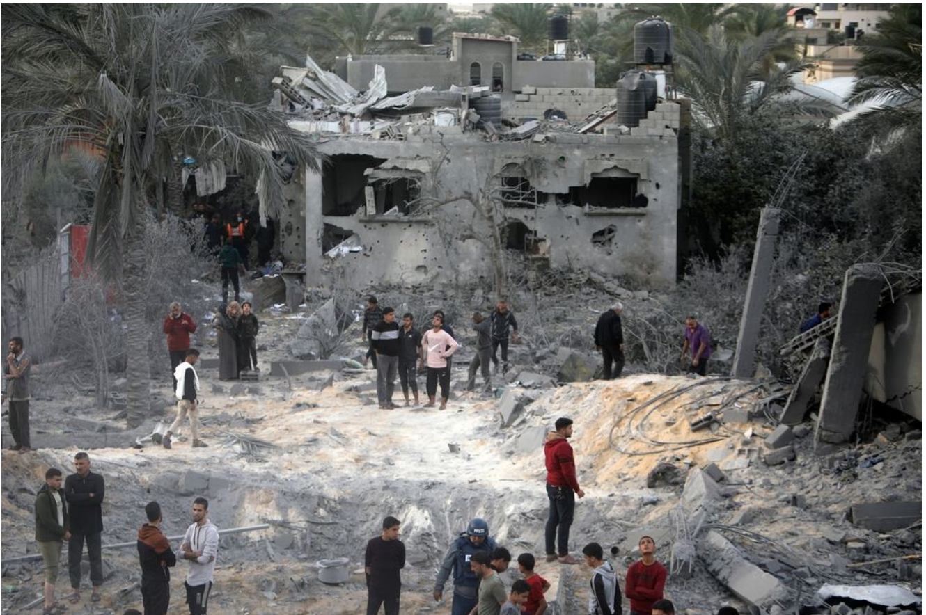
Palestinians inspect the damage of a destroyed house following Israeli airstrikes in Gaza
