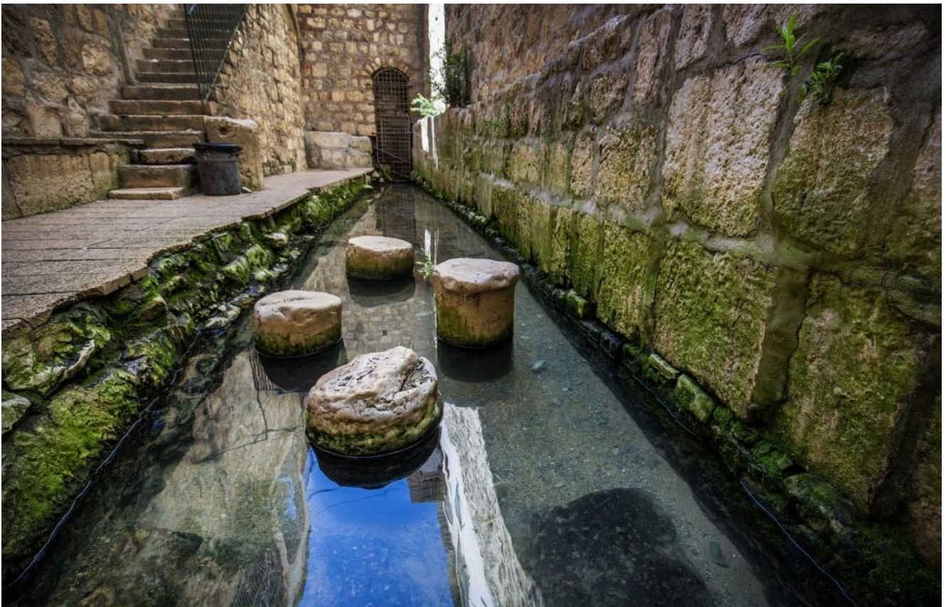
Hezekiah's Tunnel – Siloam Tunnel, Jerusalem
