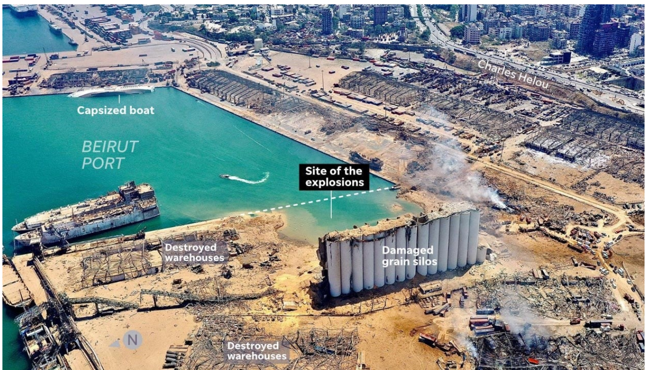
Beirut Port Damage
