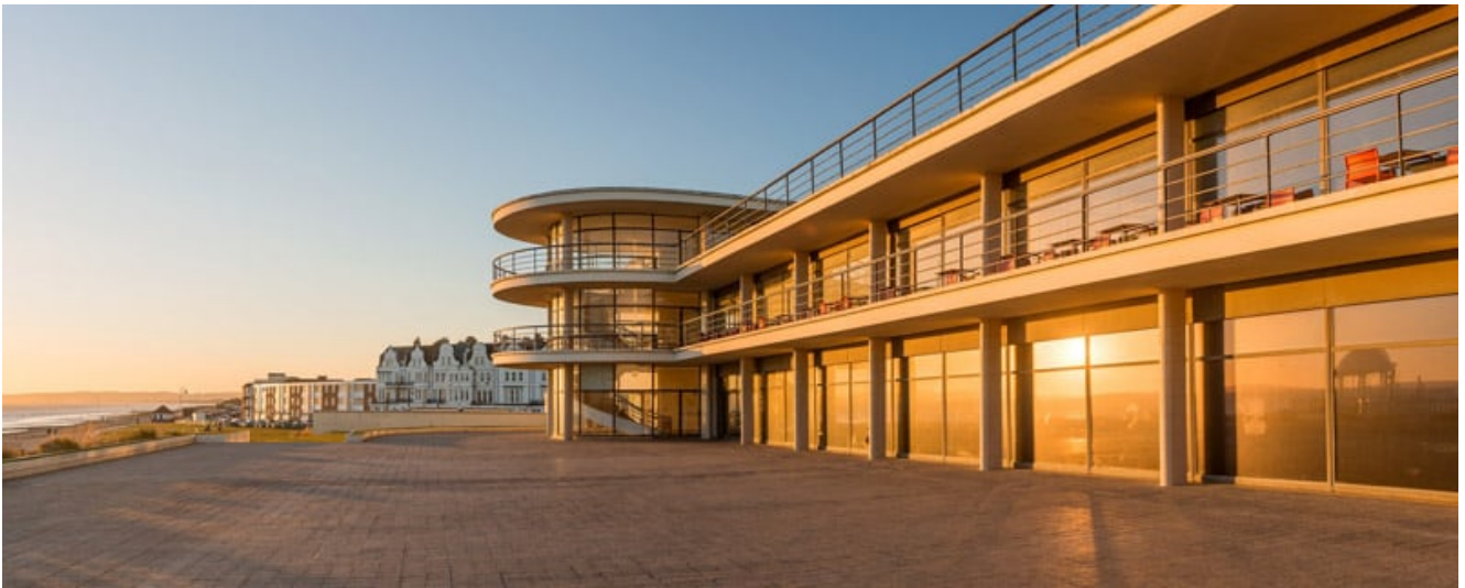
De La Warr Pavilion, Bexhill On Sea, East Sussex
