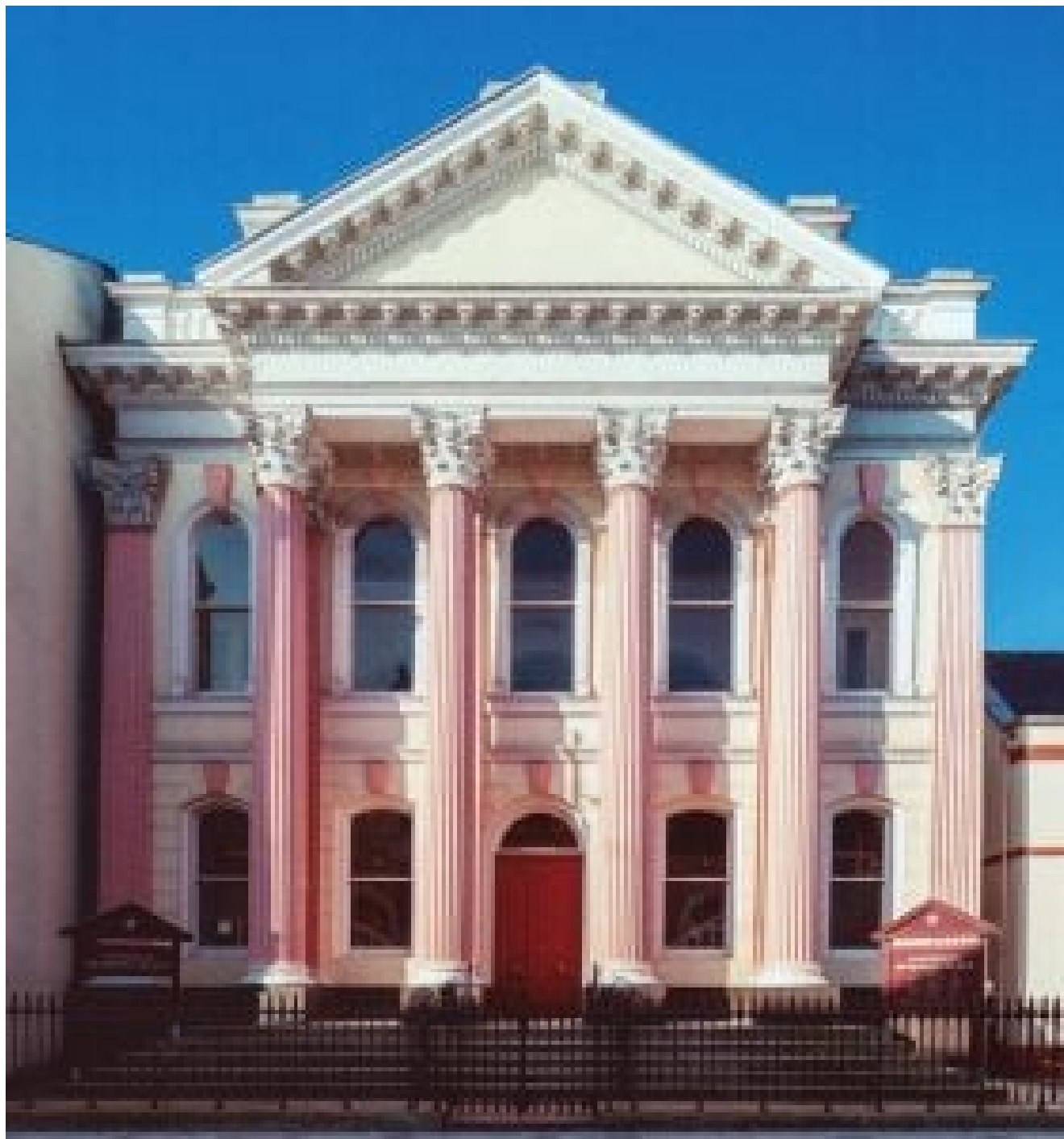
Figure 12: Confident Roman Corinthian temple-front of the Methodist Church, Darling Street, Enniskillen, County Fermanagh (1863-5).
