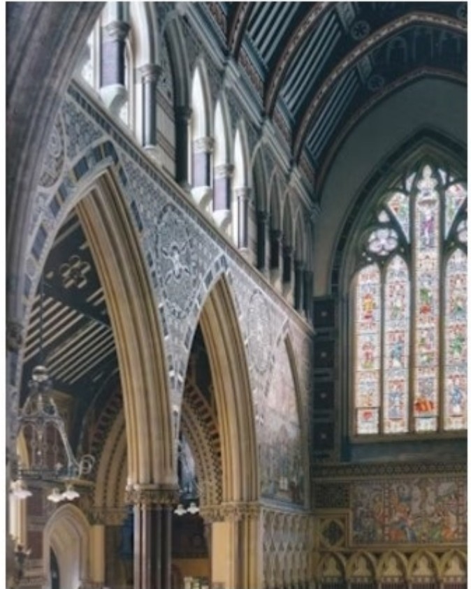
All Saints, Margaret Street, London, looking west, showing the glorious polychrome treatment of the nave arcade, the spandrels decked out with geometrical patterns, the colour in the materials used, rather than applied.
