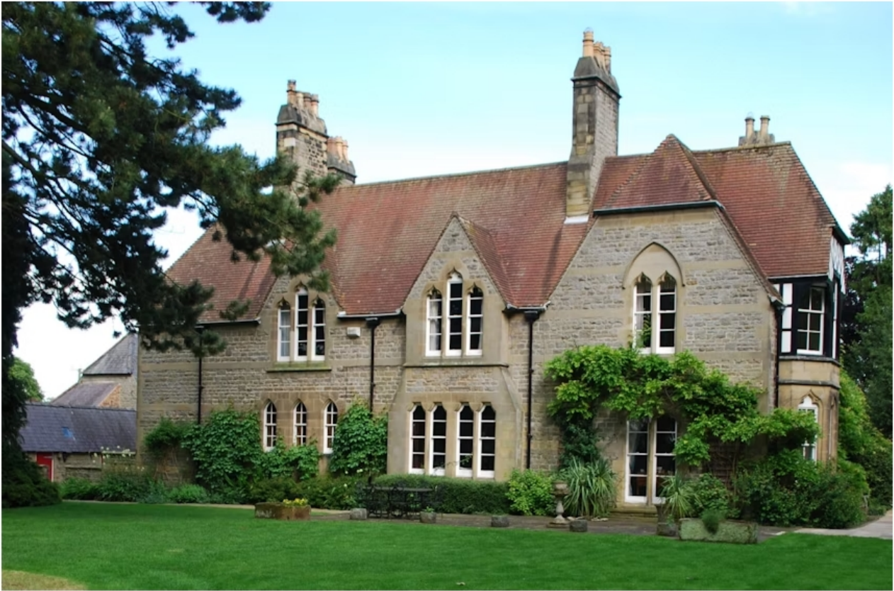
The former parsonage, north-east of the church at Baldersby St James, showing the carefully considered and emphatic Gothic detail, handled with complete assurance by the architect (© James Stevens Curl [2021]).
