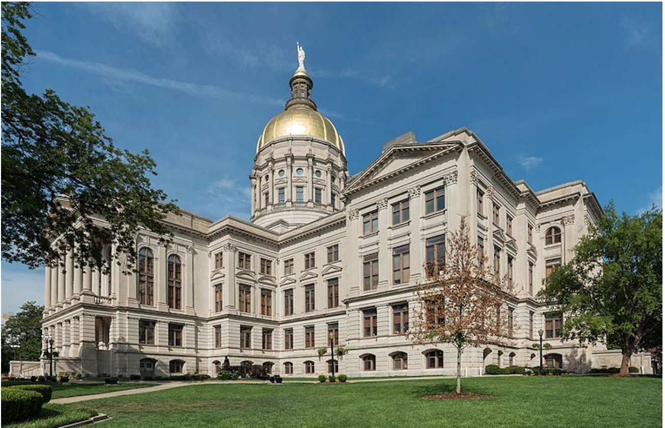
Georgia State Capitol Building
