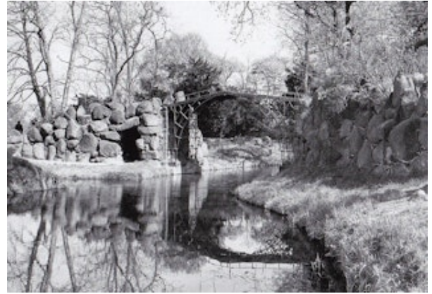
The Eiserne Brücke at Wörlitz, with rock-work abutments (1791): a scaled-down version of the celebrated Iron Bridge over the River Severn in Shropshire, designed by Pritchard and erected 1777-9 (© James Stevens Curl).
