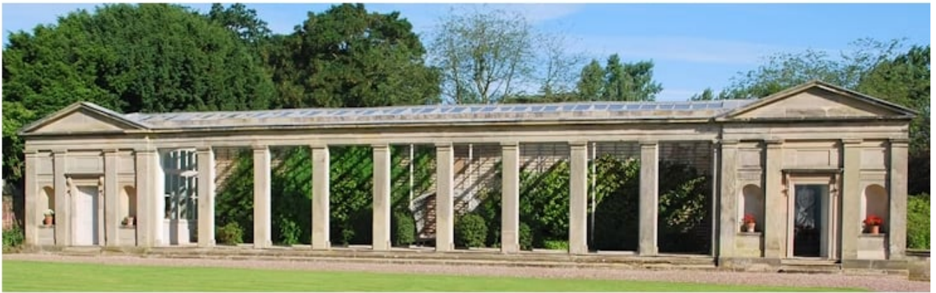
The orangery at Blithfield Hall (1769), designed by Athenian Stuart, viewed from the north range of the house (© James Stevens Curl).
