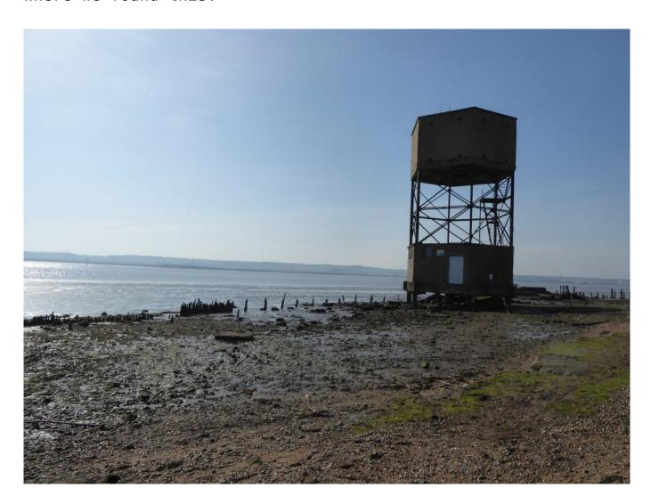
It is built to look like an ordinary water tower but that is a cunning disguise. It is (or was) a radar station, 1940-1944 placed to detect enemy submarines coming up the Thames. The crew lived in the bottom bit and the equipment was above. Some of that equipment is believed to now be in the main fort, but much was lost during the period it was near derelict.
